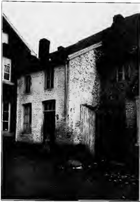
HOUSE (NEAR LIÈGE) TYPICAL OF THE WORST SLUMS.*
